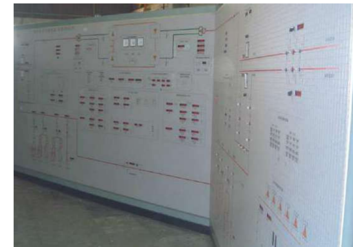
Control Panel and mimic diagrams with 48x48 tile system
